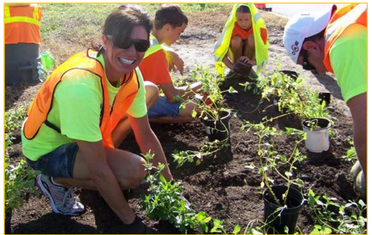
Volunteers install a "La Florida" roadside planting in Lee County.
